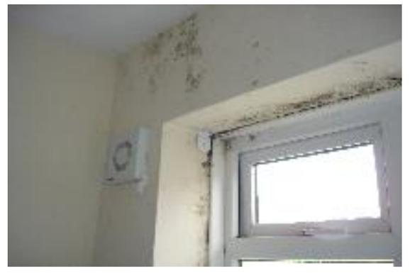
**This is typical damage we have had to attend to, caused by tenants not following advice on adequately heating and ventilating.** As this type of damage is both preventable and expensive to remedy - Homes for Life may need to recharge tenants the cost of these necessary repairs.
